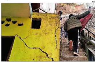
A house in Shimla shows deep cracks linked to the under-construction NHA tunnel work, and (below) families evacuating buildings
